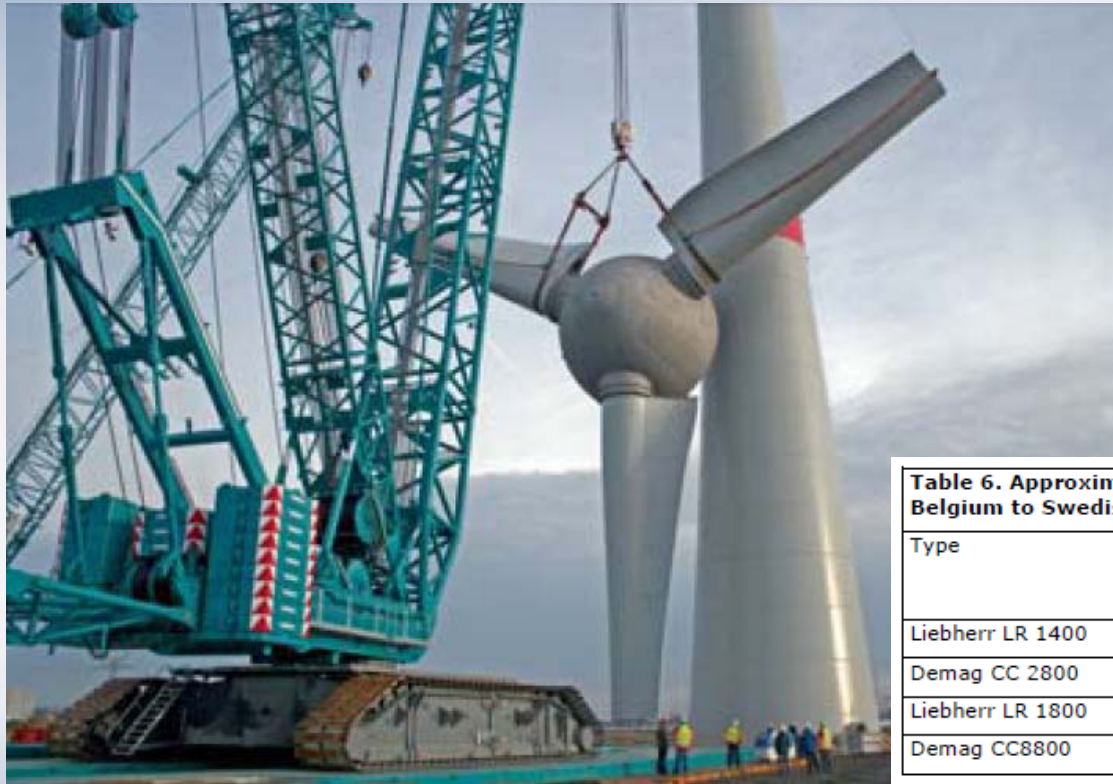
Figure 1. Lifting of the 340 t hub section for Enercon E-126 7,5 MW wind turbine. The Terex Demag CC9800 crawler crane is formally rated 1600 t and in this configuration can lift 360 t.
