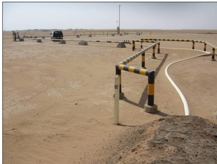
Figure 7: RTP Pipe complete joint buried and above ground lay down
