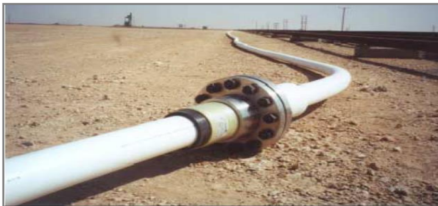
Figure 4: RTP Pipe flange coupling
