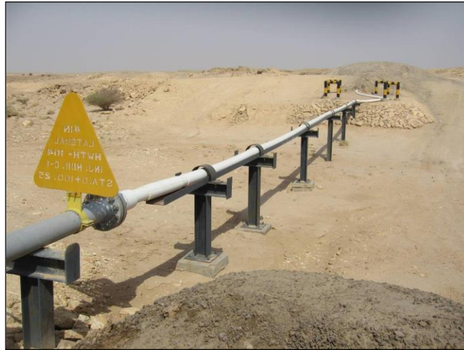
Figure 3: RTP flowline transporting water injection
