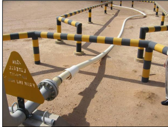
Figure 6: RTP pipe coupling to CS pipe using metallic flange connection
